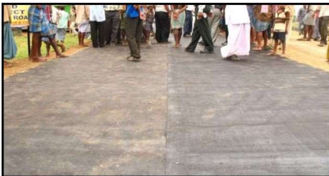
Figure: 5.4 Laying of bitumen treated jute geotextile in West Bengal
