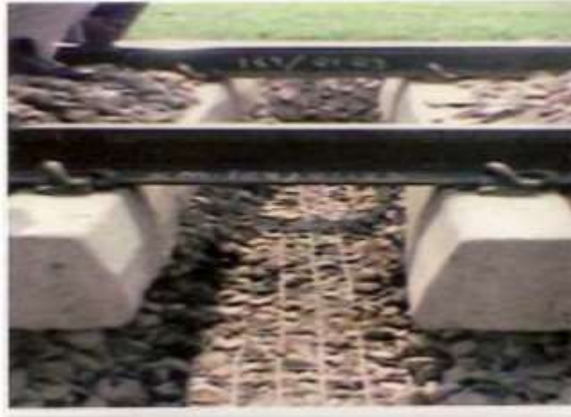
Figure: 4.3 Example of railway construction River Canals and Coastal Works:
