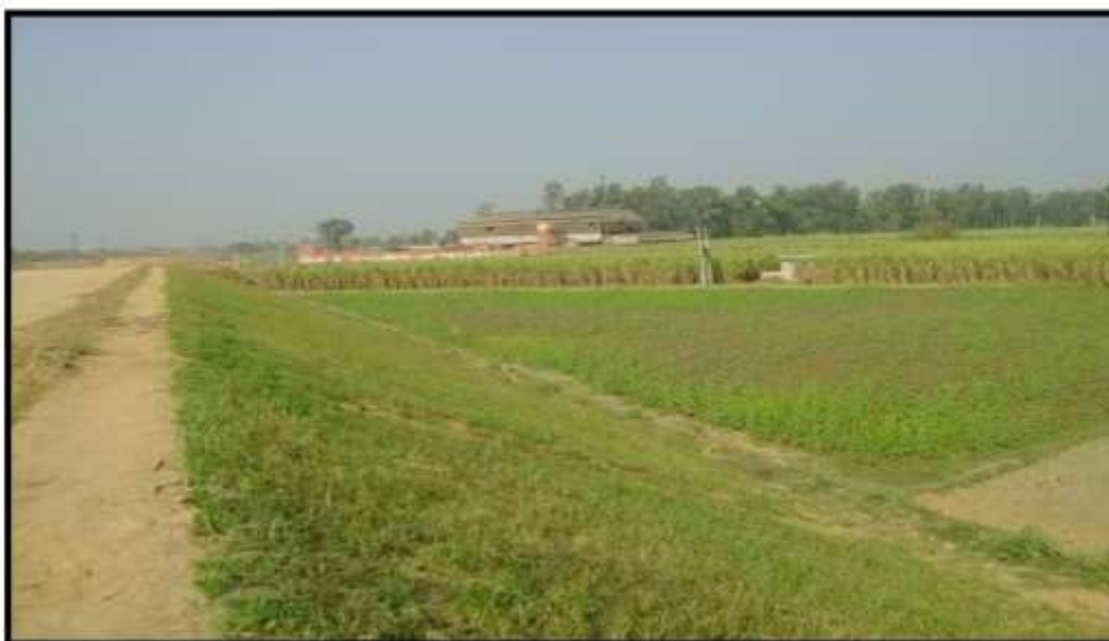
Figure: 5.4 Slope protection with Jute Geotextile
